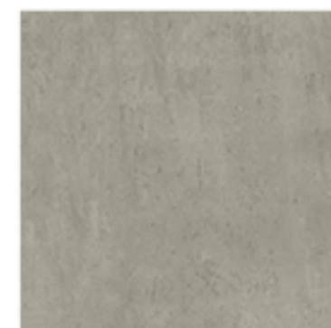
OFF SHUTTER CONCRETE FINISHES
